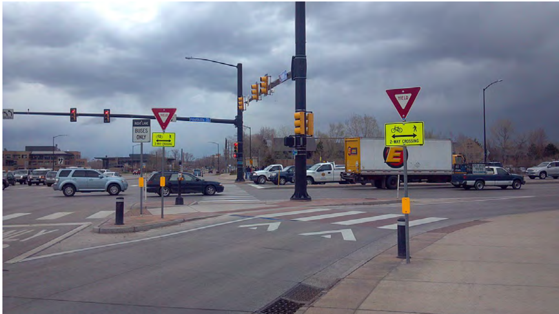
Figure 4-5 Best Practice Example: Raised Pathway Through Right Turn Slip Lane (Boulder, CO)
