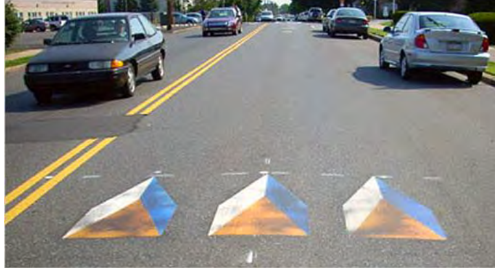
Figure 4-10 Traffic Calming Examples Using Pigmented Pavement
